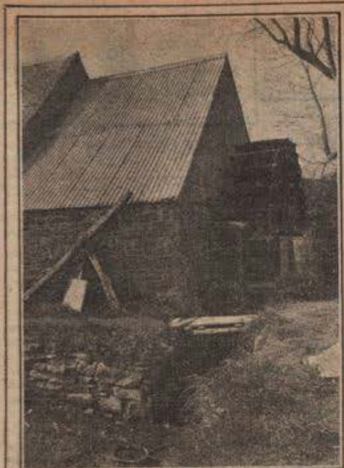
THE OLD WATER-WHEEL of the woolen yarn factory at Llanrhystyd, in Cardiganshire.
